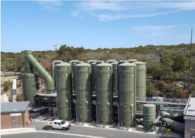
New Standby Polishing Scrubber (left), beside the Biotrickling Filter System that manages odour at the plant.
